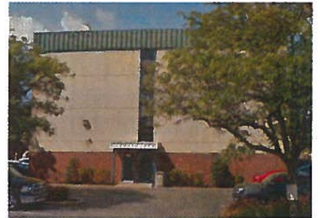
14 East Side of Building (on-site)
