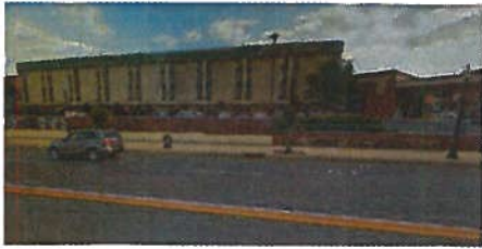
1 Across Street View - North
